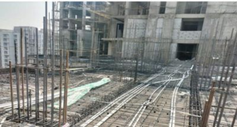
Tower - F12 - Shuttering and Reinforcement work in progress
