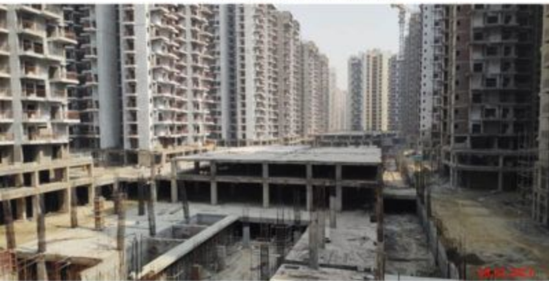
Non Tower - in between F & B Tower
