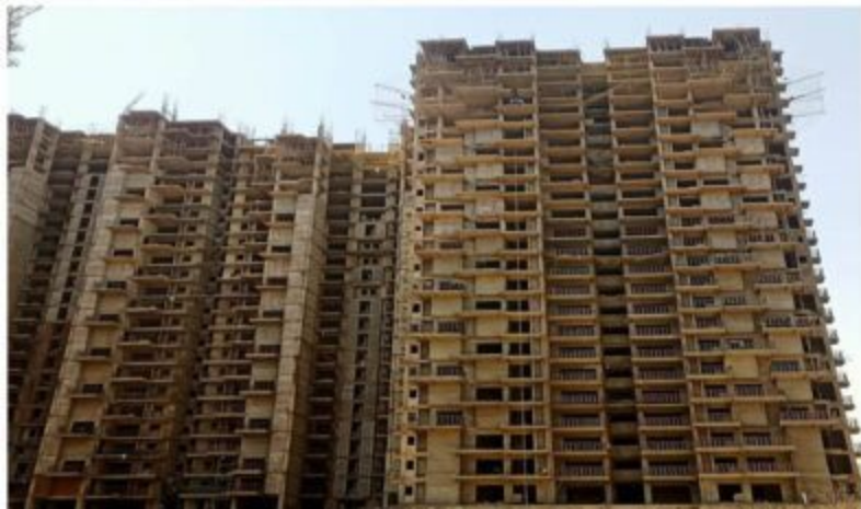
TOWER - F9 EXTERNAL PLASTER WORK IN PROGRESS
