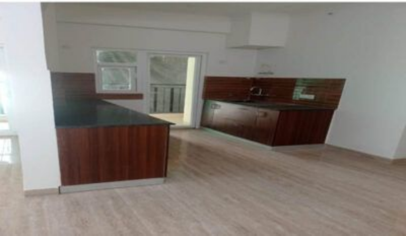
TOWER - B1 SAMPLE FLAT KITCHEN WORK IN PROGRESS
