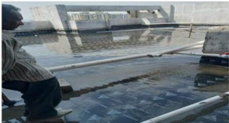
TOWER - A1 TARRECE FLOOR APP MEMBRANE WATER TESTING WORK IN PROGRESS
