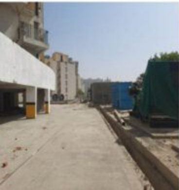
Road Work in Progress - Near O2 Valley
