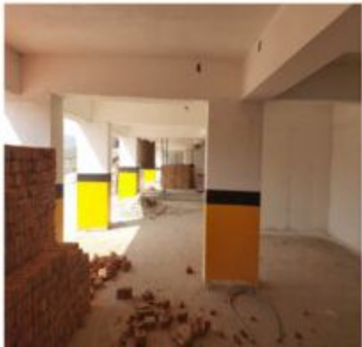
Painting Work in Progress - Stilt Floor - O2 Valley
