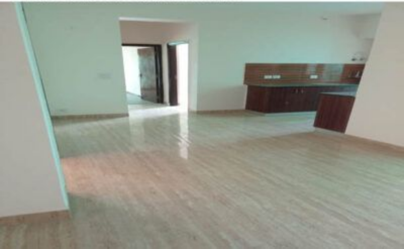
TOWER - B1 KITCHEN WORK IN PROGRESS
