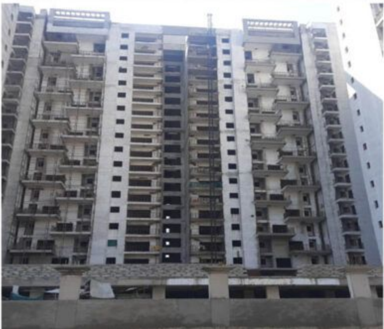
TOWER - A3 EXTERNAL PLASTER WORK IN PROGRESS
