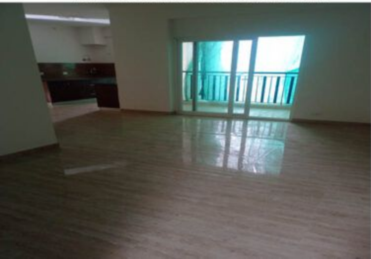
TOWER - B2 SAMPLE FLAT WORK IN PROGRESS
